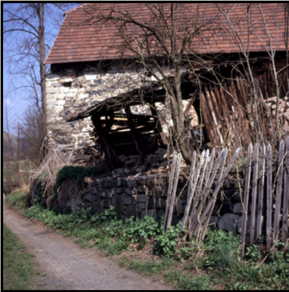
Scheune in Nordböhmen, 2005
